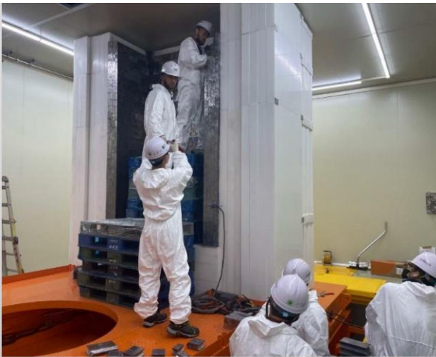
Shielding Pb and PE installation
